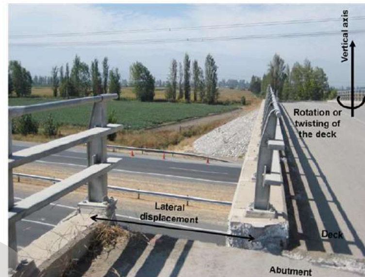
1.5 Damage to a skewed bridge after the Chile Earthquake of February 27, 2010 (source: Yashinsky et al. [2010]).
