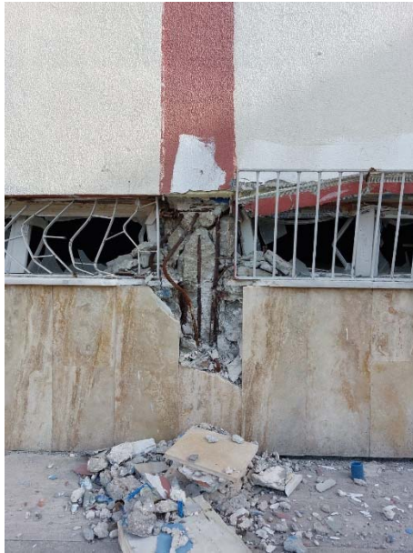
Fig. 5 Typical short-column type of damage, induced by continuous belt of low-height windows.
