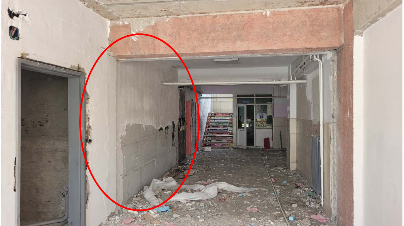
Fig. 14: Additional RC shear wall.
