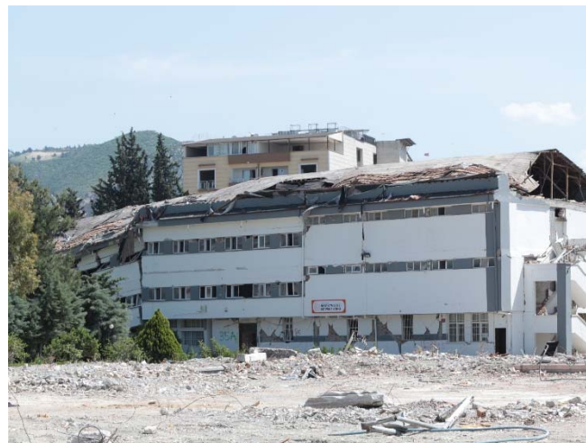
Fig. 17. Partial collapse of a large portion of a dormitory building, due to heavy damage of several consecutive columns at the ground floor.
