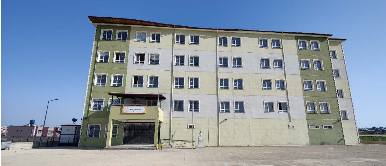
Fig. 6 – Front view of the building.
