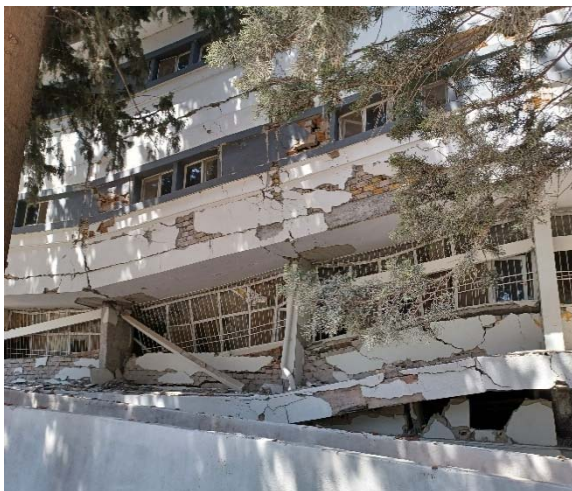
Fig. 17. Partial collapse of a large portion of a dormitory building, due to heavy damage of several consecutive columns at the ground floor.
