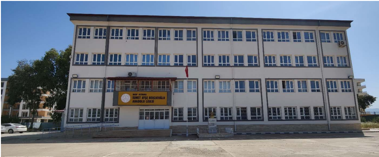
Fig. 2. -. Front view of the building.
