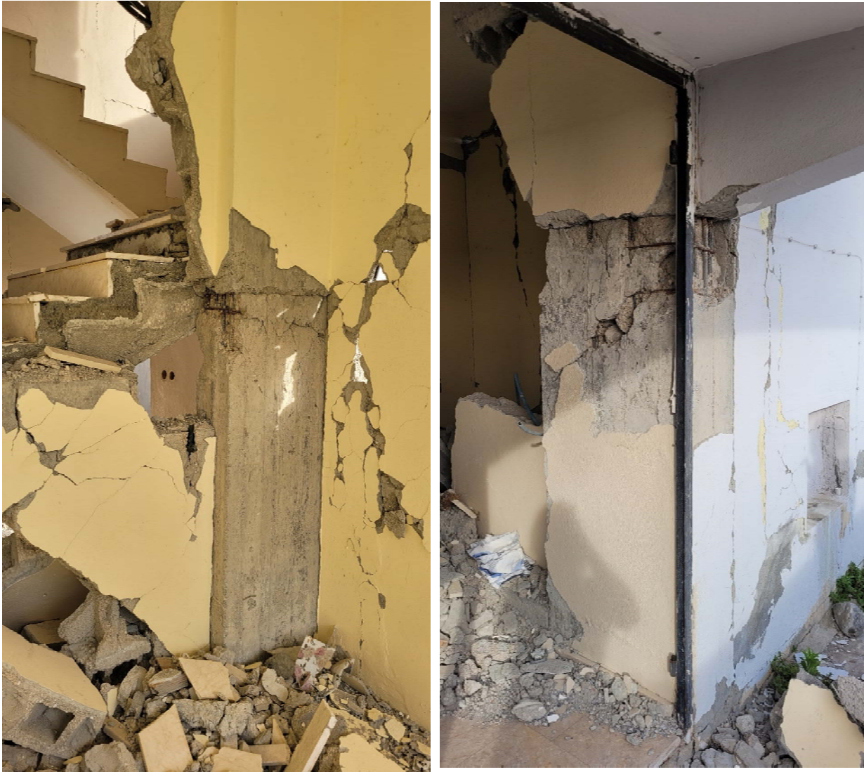
Fig. 15: Column damage
