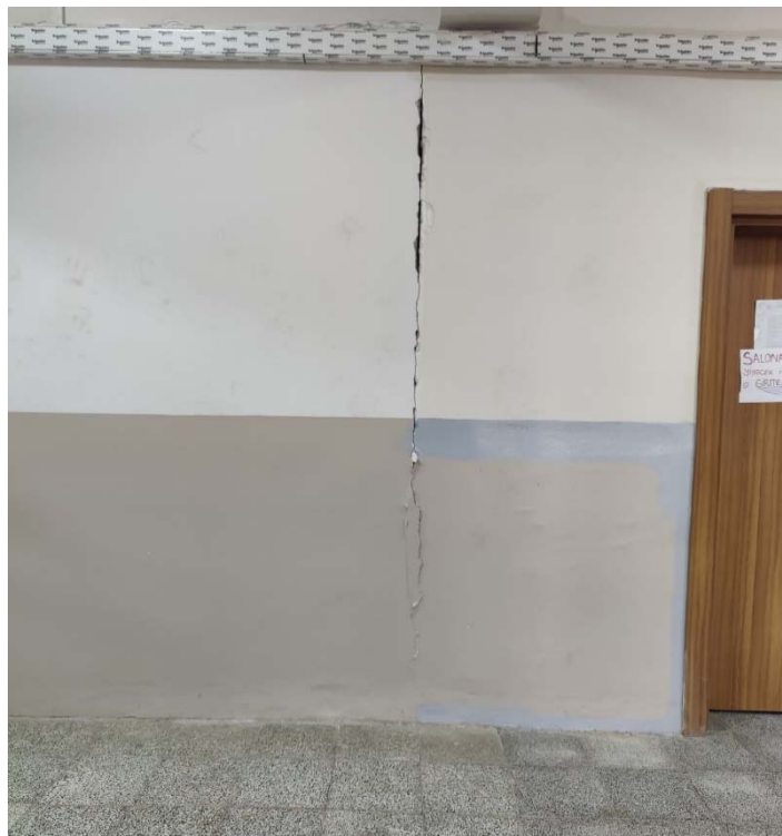
Fig. 5 – Separation of the masonry infill.
