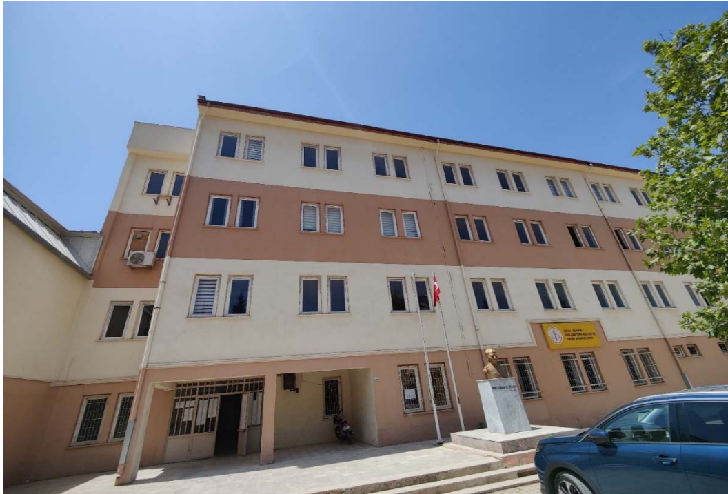
Fig. 4 Front view of the building
