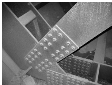
Figure 31. Bolted end-diaphragm connection detail.
