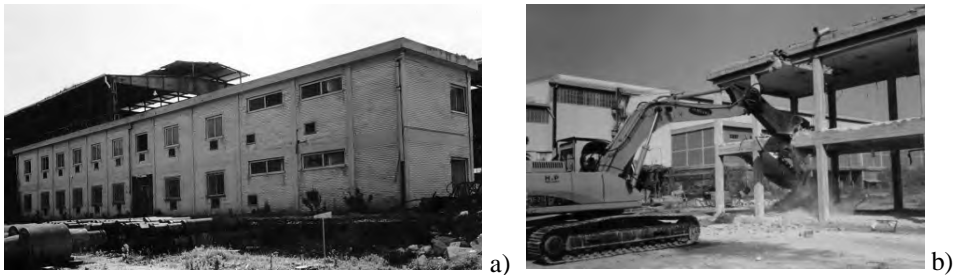
Figure 3. The building under investigation (a) and division in sub-structures (b).
