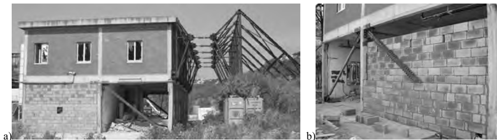
Figure 5. The tested RC building equipped with the novel BRBs.
