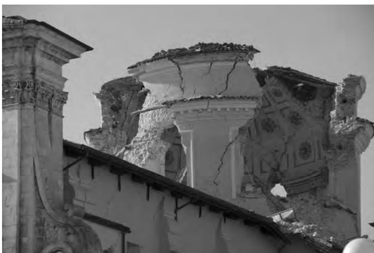
Figure 11. Typical collapse of the dome of the L'Aquila Duomo.
