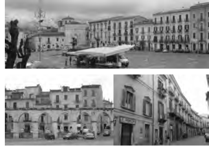
Figure 4. Masonry buildings in the historical centre of Sulmona.
