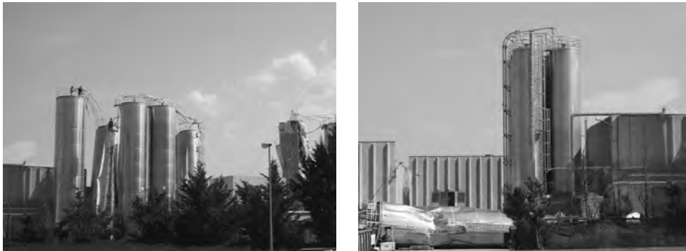
Figure 9. Damage of metal tanks between the municipality of Onna and L'Aquila.
