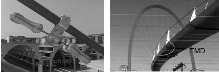
Figure 3b. TMD system.
