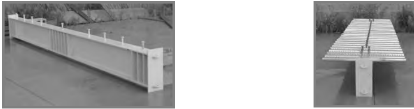
Figure 4. The beams before concrete casting.
