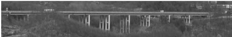
Figure 9. The viaduct “Rio Torto”.
