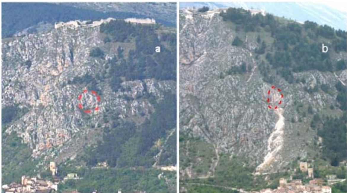
Figure 56. View of Fossa from mount Di Cerro: before (a) and after (b) the earthquake. The detachment area that generated the rock avalanche is circled. On top of the cliff (b), note the debris underneath the walls of Ocre castle produced by masonry failures.
