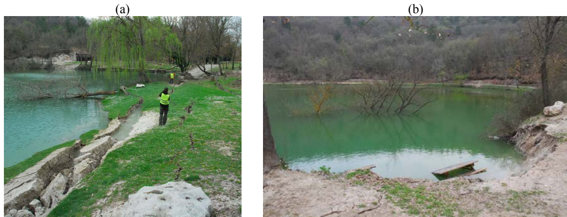
Figure 60. Fractures along the NW perimeter delimiting slices and blocks lowered and rotated inward (a). Lowering of a large block detached from the western margin, evidenced by the submerged trees (b).
