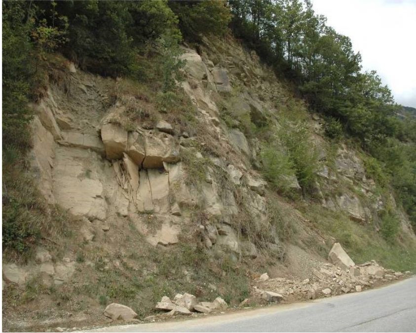
Figure 4.6. Free-face wedge sliding that is governed by bedding joint attitude.
