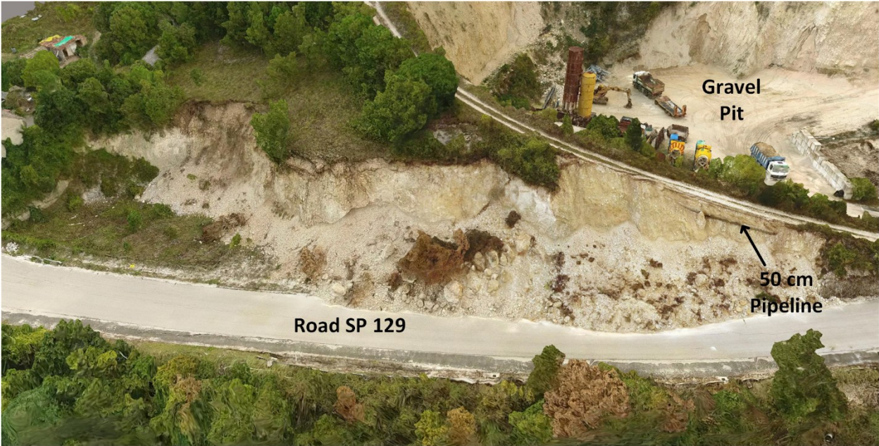
Figure 4.36. Model image of landslide near gravel pit and Road SP 129 that exposed a 50 cm-diameter pipeline (42.74950 N 13.26958 E).
