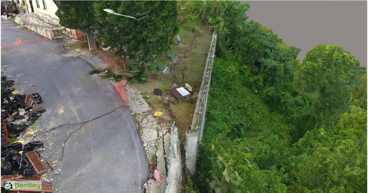
Figure 4.43. Rotated retaining wall and subsequent graben behind the wall. Soil settlement between 45-50 cm behind the wall, and formed cracks up to 45 cm in width (42.69446 N 13.24980 E).
